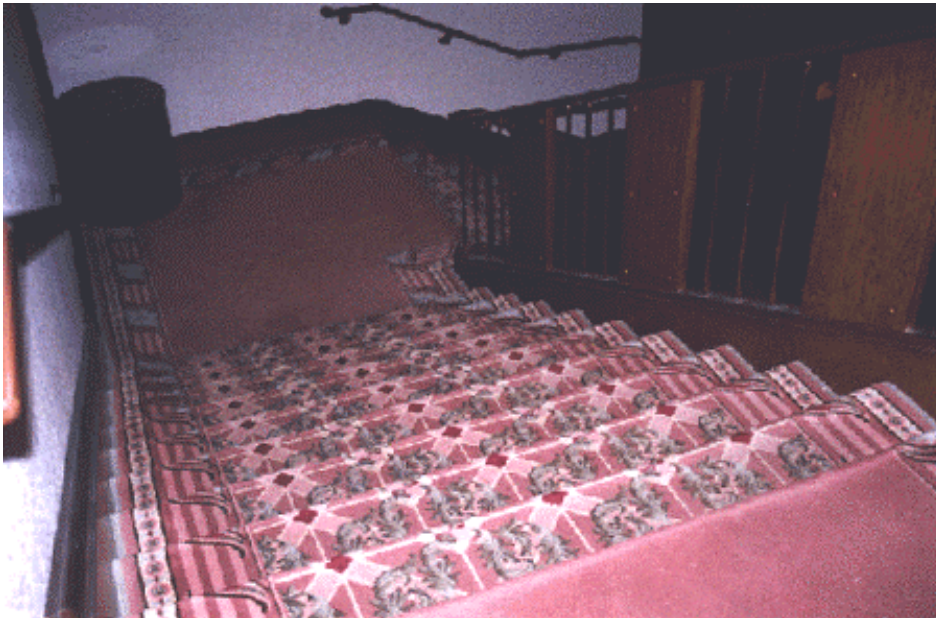
Figure 1 Vivid carpet patterns on stairs create special perceptual problems for the elderly.
